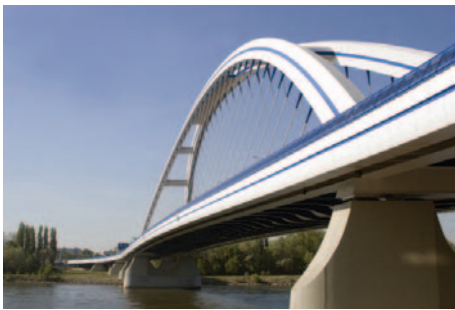
Apollo bridge, Bratislava
